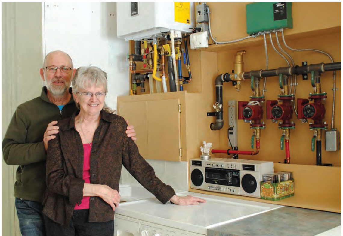
► Tom and Dee Ashman in the laundry room near the household mechanical systems that provide on-demand domestic hot water and back-up heat through in-floor heating.
